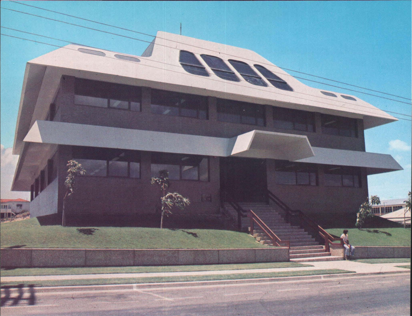
TRANSPORT— Chapter 14 Gladstone Harbour Board Offices
